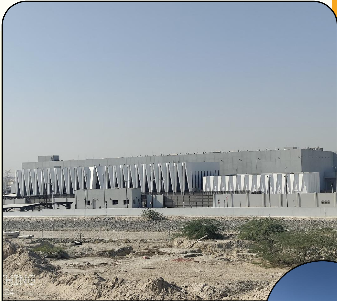
Khazna Data Center DX03 – IBN Dubai
